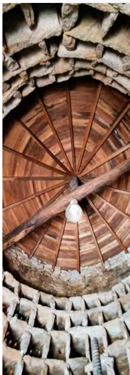
Vista interior cuberta restaurada
